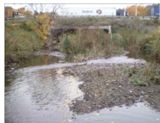
Existing twin cell culvert at Fletcher's Creek
